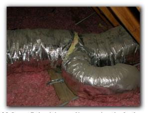
25. Loose fitting joints and/or openings in the ductwork should be sealed. This item should be repaired to increase the efficiency of the system. Repairs are fairly easy, and approved supplies/materials are available at most big box home stores.
