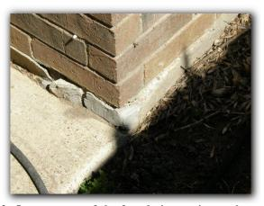
2. One or more of the foundation perimeter beam corners were observed to be sheared off (corner pop). This is a common condition in slab on grade foundations. This condition does not adversely affect the performance of the foundation. However, in some cases, some cosmetic improvements may be necessary.
