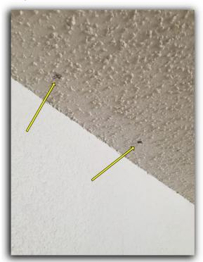
10. There are "nail pops" on the ceilings and/or walls in one or more rooms of the house. Nail pops are caused when the heads for sheet rock nails push through the interior finish. These are easily driven tight and patched.
