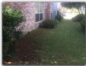
3. The grading should be improved to direct storm/rain water away from the house. This can usually be accomplished by the addition of top soil. The ground should slope away from the house at a rate of one inch per foot for a minimum of ten feet. Ideally, at least eight (6) inches of clearance should be maintained between soil level and the top of the foundation walls.
