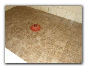
The shower pan was tested by filling it with 2 inches of water and inspecting for leaks around the exterior walls of the shower pan. I did not observe any indications of leaks at the time of this inspection.
