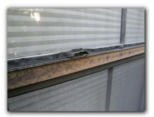
14. Exterior weather stripping on the Den windows has degraded or is ineffective. Loose or improperly secured glass panes are considered a recognized hazard. Proper weather stripping the windows will also make the house more energy efficient and quiet.
