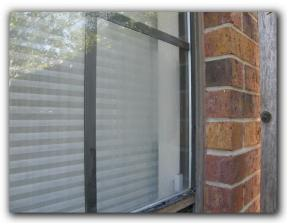
13. One or more of the thermal pane windows in the Master Bedroom, have lost their seals. This causes condensation or a fog like film to develop between the panes of glass. These windows loose their insulating properties and replacement may be necessary.
