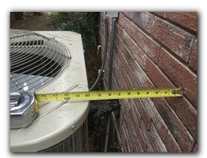
24. <u>The outside condenser/coil is set too close to the house.</u> Current standards recommend a minimum of 12" to allow sufficient air flow and efficient operation.
