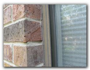
15. The majority of windows need caulking repaired/replaced at the brick/ siding, or trim. Repair of this seal will stop water infiltration, and possible damage to the structure and/or finishes. Recommend using an elastomeric caulk, available at most big box home stores.
