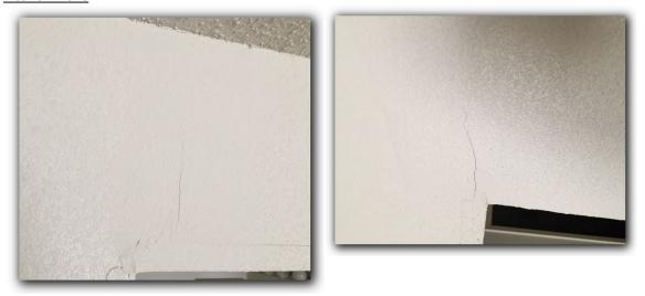
7. Common hairline cracks were noted in the interior gypsum wallboard, in one or more locations. Cracks near the interior windows and doors are usually indications that there is some degree of movement occurring in the structure. It is normal for any structure to have some degree of movement. This is typical for this area, and is not a big concern.
