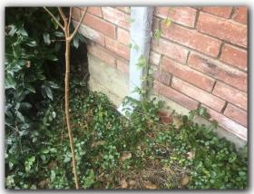
4. <u>One or more of the downspout extensions are too short.</u> The gutter downspout's should discharge water at least 3-feet to 5-feet away from the structure. Storm/rain water should be directed to flow away from the building at points of discharge.
