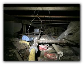
1. <u>Crawl space has debris in one or more sections under the house.</u> This debris allows rodents and other varmints to exist under structure. Debris should be removed and a clean environment maintained.
