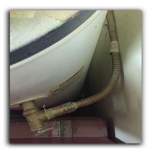
29. The discharge pipe for the temperature and pressure relief (T&PR) valve has been downsized. Current building standards require the discharge pipe to be the same size as the outlet of the valve, and cannot be reduced at any point, have any kinks or restrictions in the pipe, or have a threaded end. (Note: a flex line is considered a reduction in size). Recommend repair by a qualified, licensed plumber.
