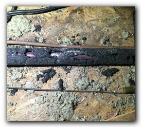
Damaged, deteriorated and/or missing insulation on the refrigerant lines in the attic area should be repaired or replaced as necessary.
