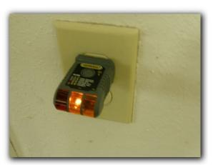
22. One or more receptacles in the Office, appear to have an open ground connection. This receptacle(s) and circuit should be further investigated by a qualified, licensed electrician, and repaired as needed.
