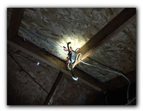
20. Improperly spliced and terminated electrical wires were observed in the attic area, located over the *Hallway*. Spliced wires in the attic should be properly enclosed in junction box(s) with appropriate covers, and secured to the rafter. This is a fire and safety hazard.
