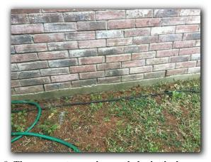
8. There are not enough weep-holes in the lower course of masonry veneer, on the West, East side of the house. Under current building standards, there should be weepholes in the lower course of the
