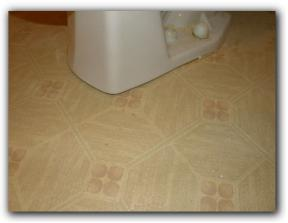
27. <u>The commode is not sealed to the floor.</u> Under current building standards the commode/toilet should be caulked to the floor around the perimeter of the base. This condition should be corrected..
