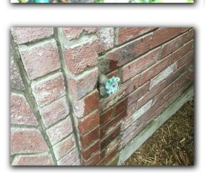
26. One or more of the exterior hose bibb(s)(faucets) do not have back flow preventers. Anti-siphon devices (Vacuum Breakers) keep contaminated water from entering the potable water of the house
