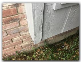
9. The exterior trim and/or siding has areas of soft/damaged, or decayed wood, at the Northeast side of the house. Recommend replacing all deteriorating/ damaged wood.
