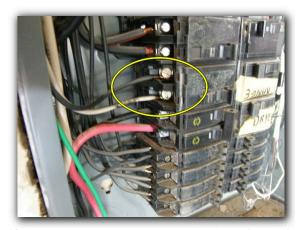
18. There are one or more Black (hot) and/or White (neutral) wires incorrectly labeled. Under current electrical standards; A Black (hot) wire used as a neutral must be labeled with white tape. A White (neutral) wire used as a hot, must be labeled with black tape. Recommend further evaluation by a qualified, licensed electrician, and repairs made as needed. It appears there may have been black marking tape on this wire at one time, but was removed or has fallen off. It should be replaced.
