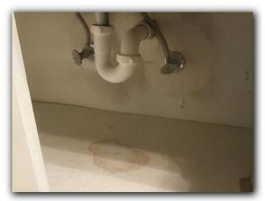
28. There is a leak in the P- trap under the Guest Bath sink. These leaks can allow water penetration to the surfaces and/or structure. Concealed damage is a possibility. The P-trap should be serviced and any damaged components replaced or repaired.
