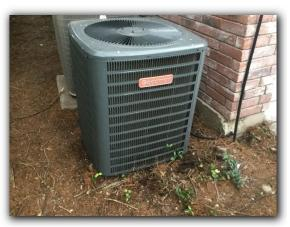
23. The Heat Pump outside condenser/coil does not appear to have proper clearance above the finish grade (ground). The outside unit should have a minimum of 3-inches of clearance above finish grade (ground). This condition should be corrected to help prevent damage to the unit.
