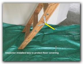
6. The attic pull down ladder steps have been cut too long. All sections of the ladder should be in line when fully extended. The lower section of steps should be trimmed so the hinge joint completely closes when in use. This situation puts undue stress on the hinge joint, and could fail when in use. This is a safety concern, and should be repaired as soon as possible.
